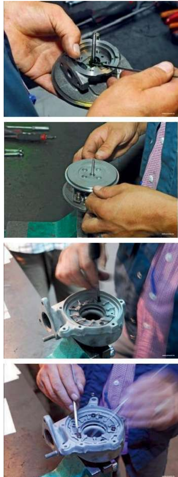
Figure 17. Reconditioning of turbine parts [1]
